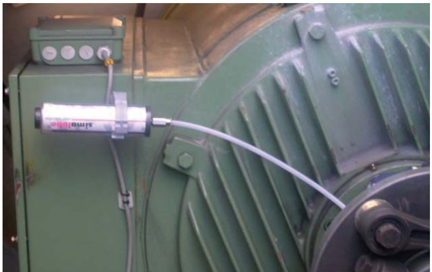
Lubrication of the generator.
